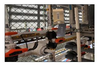
IWD-9: Sampling connection in AWN weir after the CH8 AWN treatment system (Metal Finishing Compliance Point for CH8 facility)
