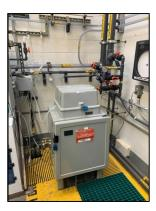
IWD-5: pH Neutralization tank of the CH6 AWN System (Metal Finishing Compliance Point for CH6 facility)
